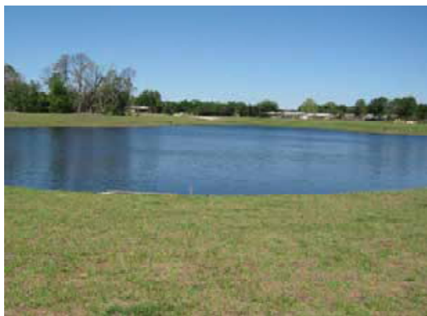
C-7 Canal wet detention pond
