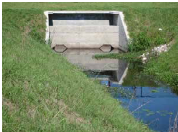
Pond discharge to C-7 Canal
