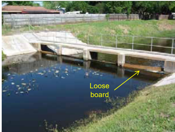
a. Control structure on upstream side of canal
