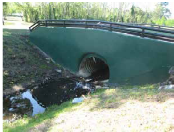
Culvert crossing at Delores Drive
