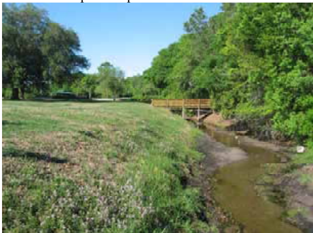
Canal downstream from pedestrian bridge
