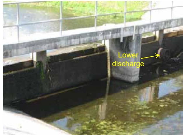
b. Control structure on downstream side of canal
