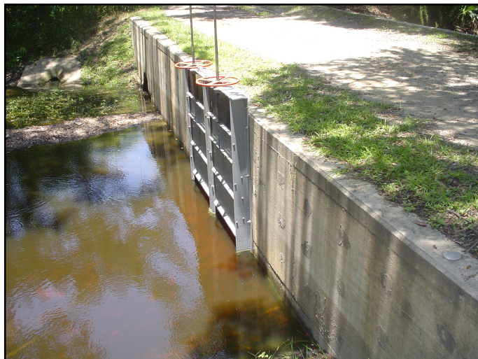
Primary Outfall Structure
