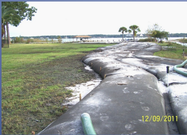
Recycling of canal sediments using geofilter tubes
