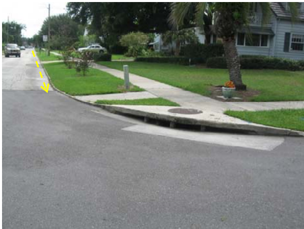
a. Curb inlet at end of Ohio Street
