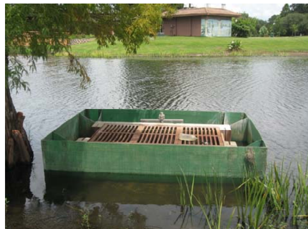
b. Outfall structure to Lake Killarney
