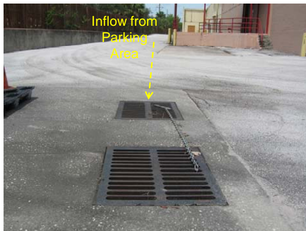
a. Final grate structures of stormsewer system
