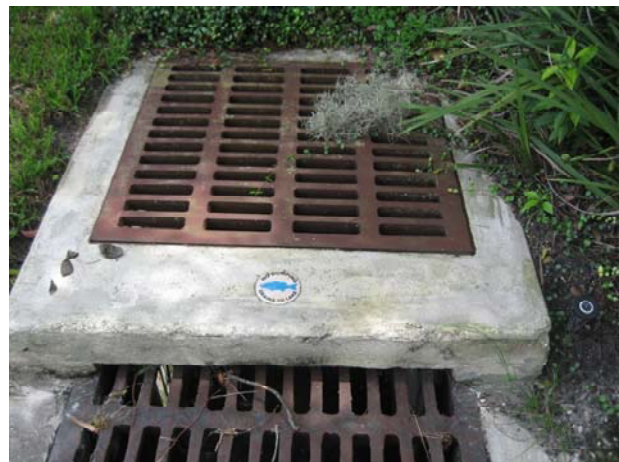
b. Overflow grate with "Drains to Lake" decal
