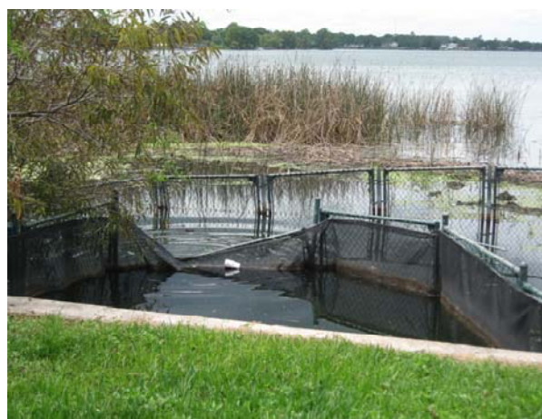
b. Leaf and debris trap at pipe outfall
