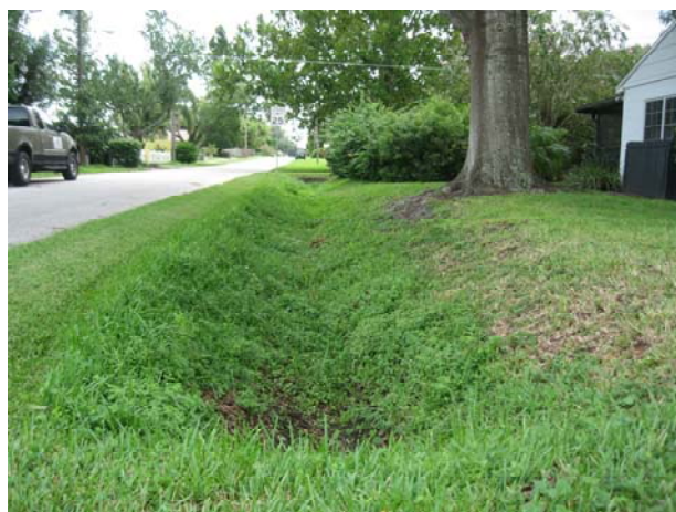
a. Typical swale drainage system along Formosa Ave.
