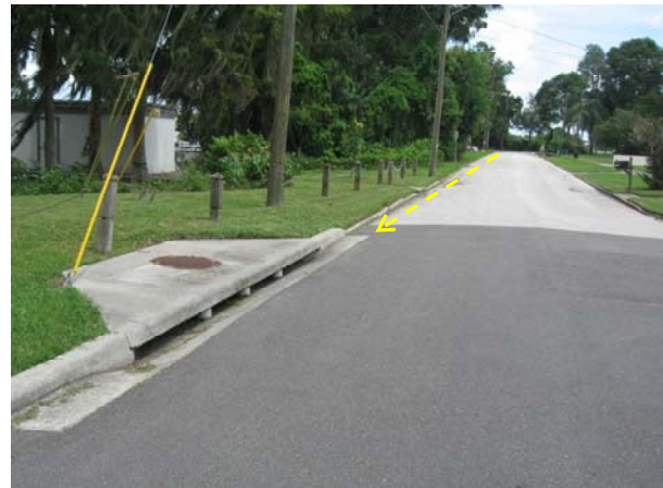
b. Curb inlet on Killarney Drive
