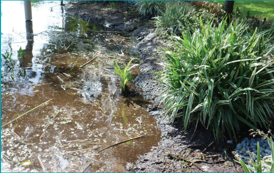
Shoreline erosion due to wave action.
